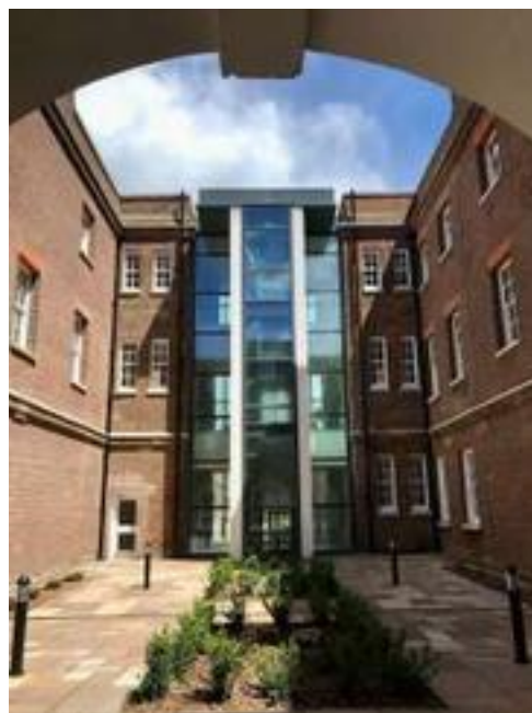
South wing converted Celia Clark 2024
