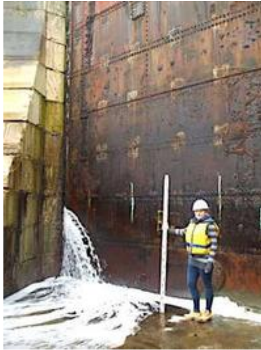
Leaking caisson
