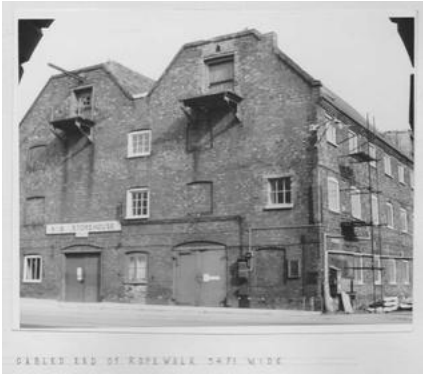
Ropery in 1956: Attic storey demolished; internal floors removed Deane Clark
