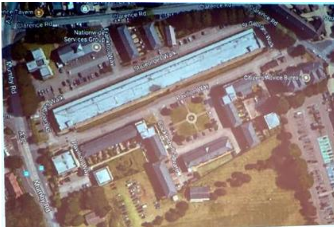
St. George Barracks redeveloped.
