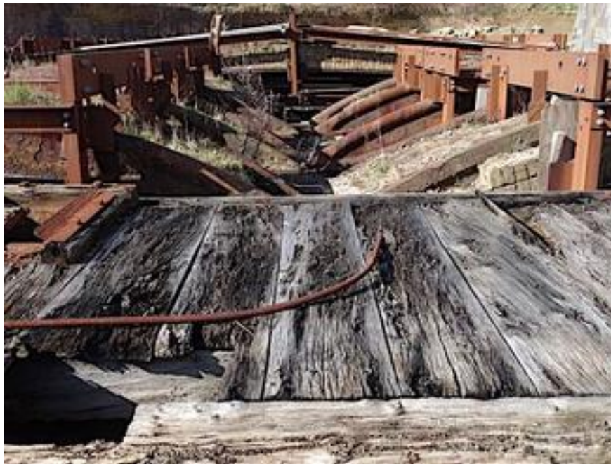
IK Brunel's 1809 bridge in Fort Cumberland. Celia Clark
