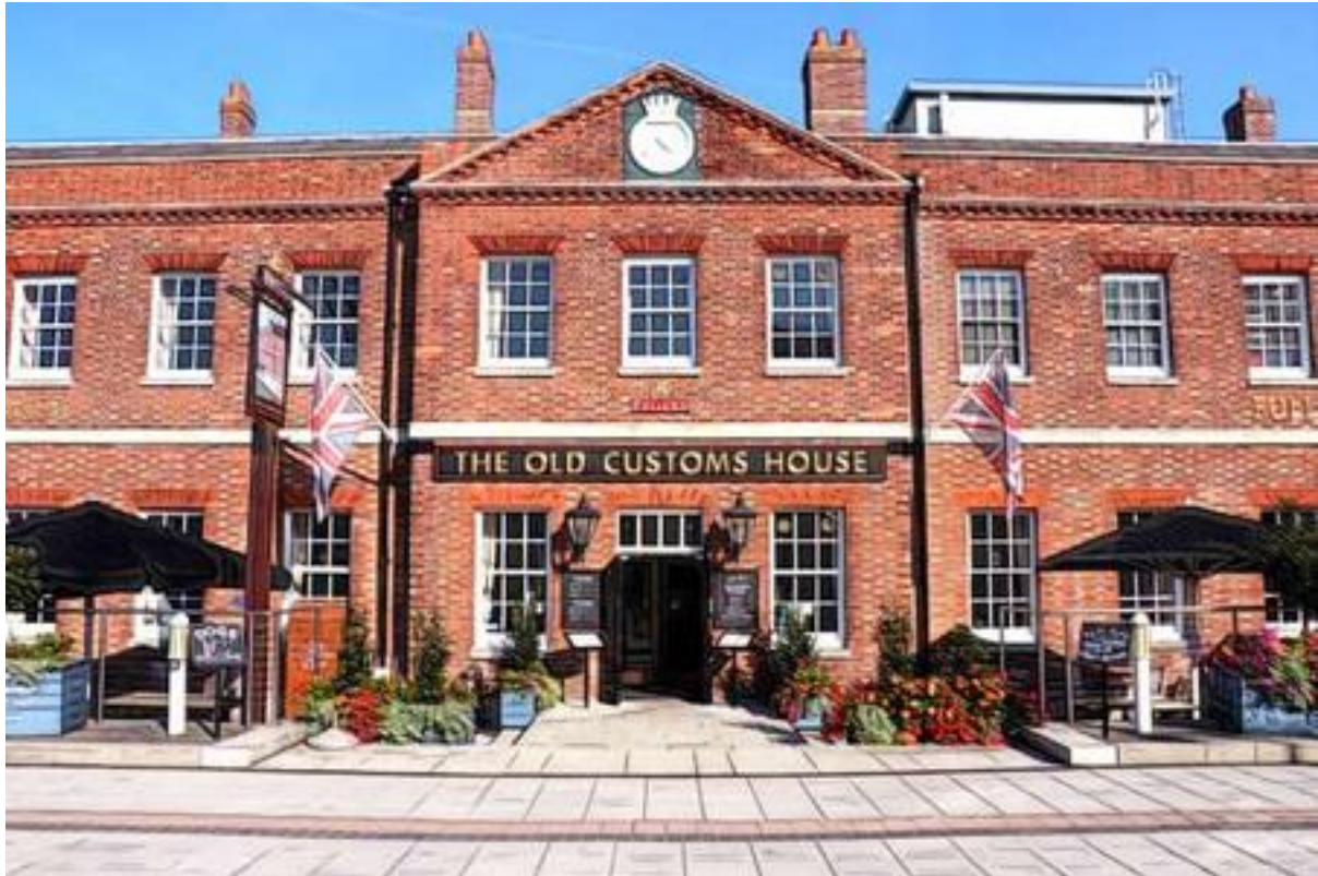
Customs House pub Gunwharf
