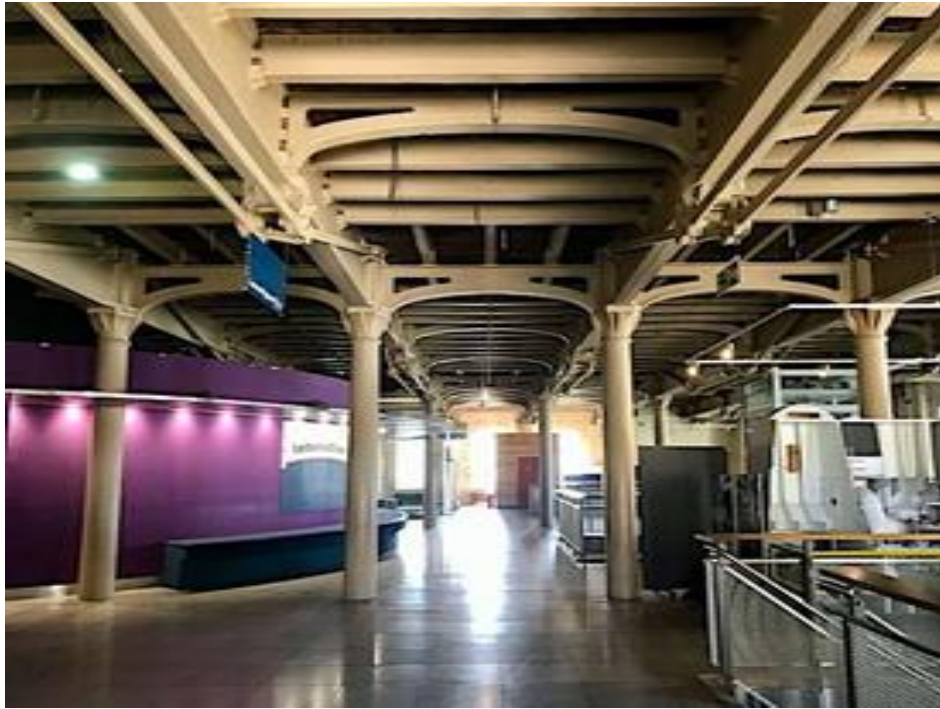
No. 6 Boathouse Portsmouth dockyard Heritage Area
