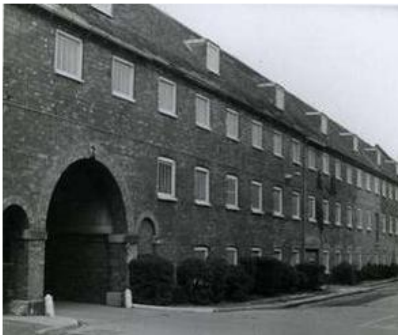
Ropery south façade
