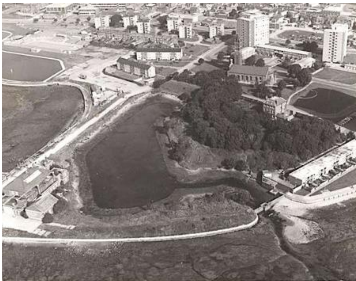
Gosport Lines Bastion No.1 before restoration. Gosport Borough Council
