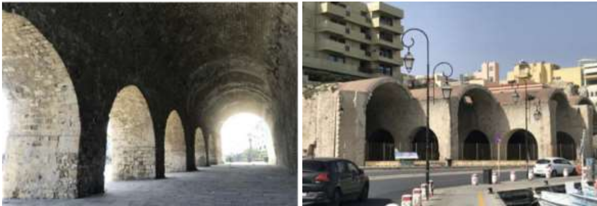
Construction of the promenade and expansion of the port led to demolition of many of the shiphalls. Only four half-length vaults of the Vechi and five of the Nuovi survive.
